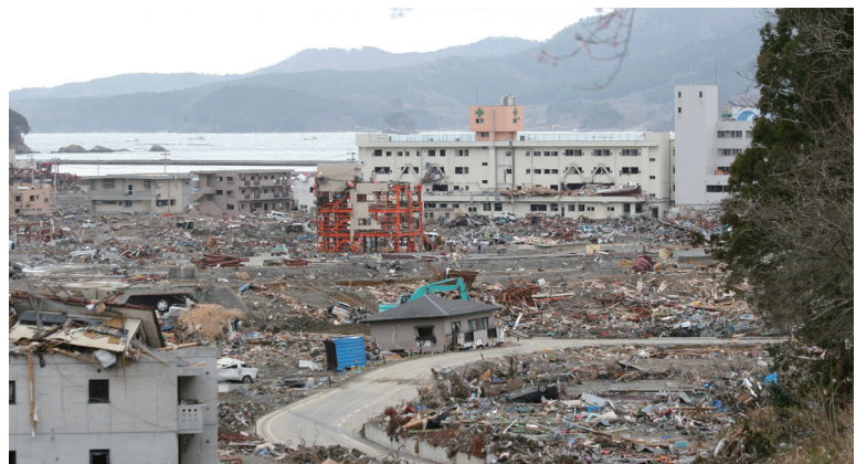
Tsunami damages during the Great East Japan earthquake. Minamisanriku in Miyagi Prefecture © Christopher Johnson
